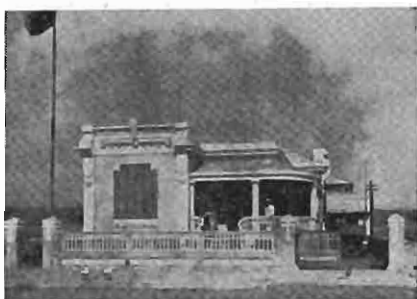
In this picture we have a view of the transmitting building and antenna system of CR6AA. The building is beautiful and the equipment modern.
