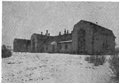
From this building come the signals of HAL, HAS3 and HAT4. It is located in Szekefehervar, Hungary. The photograph is furnished by J. Muranyi, 27 N. Highland Ave., Akron, Ohio. The programs of these stations are eagerly sought by Americans of Hungarian origin.
